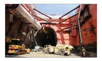
Figure B – Large area excavated for an underground LRT station<sup>2</sup>
