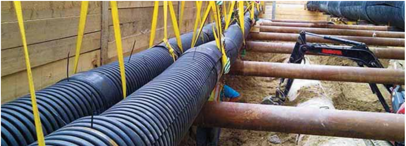
Utility Coordination Efforts on the TTC Union Station Expansion Project
