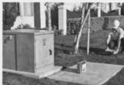
Electrical Inductive pinpointing of electrical cable.
